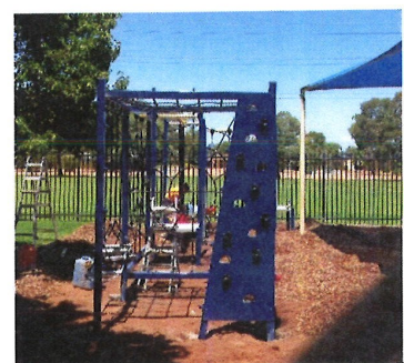
Here is the climbing frame and being built.
